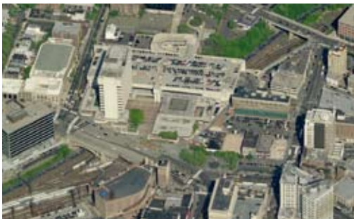
The Journal Square Transportation Center at the PATH Plaza (center right) is at the heart of the Journal Square study area.
